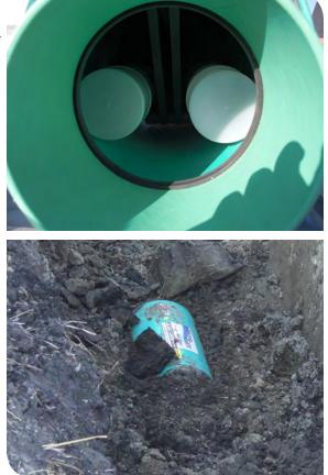
Automatic water control valve (in place)
