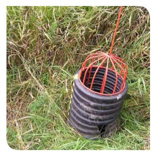
Figure 14. Standpipe side inlet in Kandiyohi County, MN.
